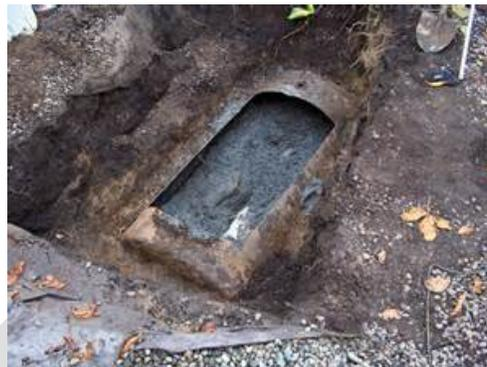
*Water Quality Concerns:* Underground storage tanks (USTs) are used throughout Rhode Island to store petroleum products such as motor fuels and heating oils and to a lesser degree other types of chemicals. UST facilities have potential to cause significant pollution of groundwater should a leak or spill occur.
